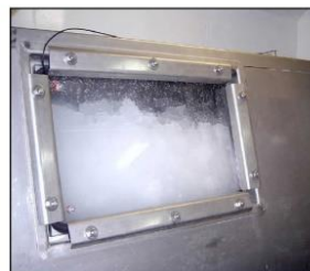
Thick Multi-Ice at 40% concentration stored in a insulated buffer tank.
